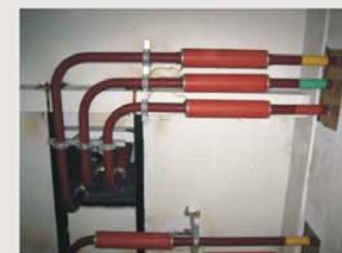
用于户内架空布置安装效果 Applied to layout of indoor overhead installation
