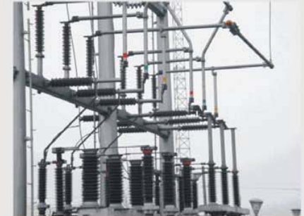
用于敞开式组合电器连接母线 Applied to open type GIS busbar connection
